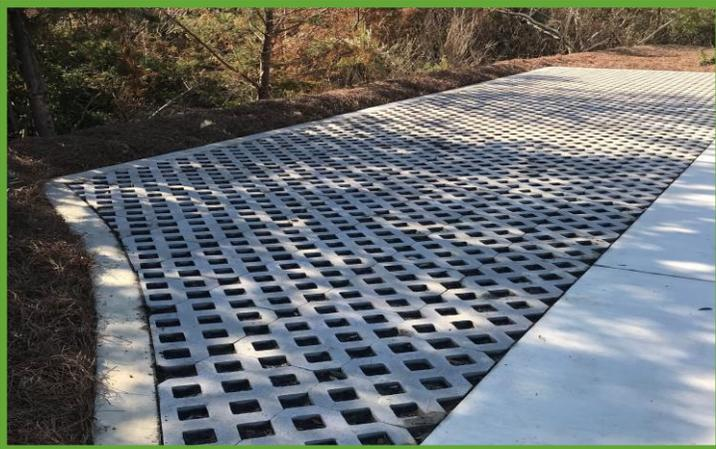
Another ecological feature of the project is a pervious pavement parking area, seen to the left. The client could have chosen to use an impervious material, but their commitment to the environment was enough to justify the extra expense. In this case, we used Turfstone which will be covered by turf eventually and look like part of the lawn.
